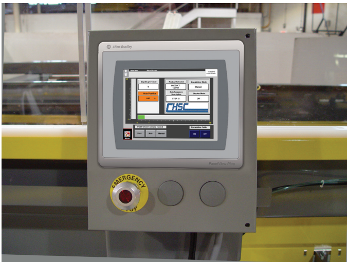
Allen Bradley controls
